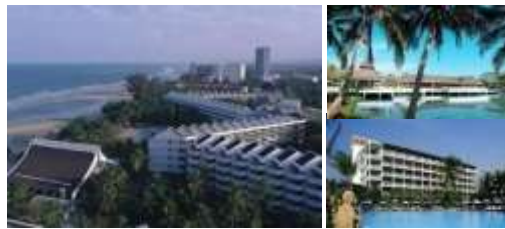
HOLIDAY INN REGENT BEACH CHA-AM (Renovation) - M.E.P. -
