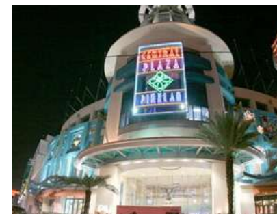
CENTRAL PLAZA PINKLAO (The Renovation) - M.E.P. -
