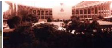
HUAMARK STADIUM - E -
