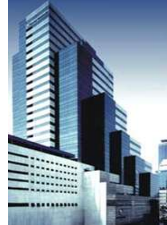
SILOM COMPLEX -E,P-
