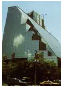
SIRIPINYO BUILDING - M,E -
