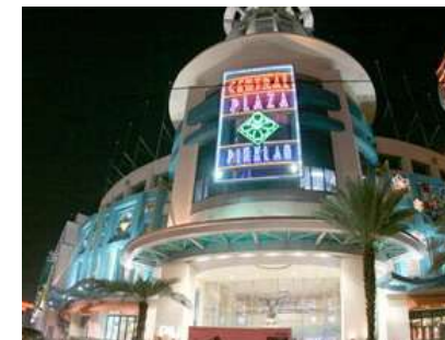
CENTRAL PLAZA PINKLAO (The Renovation) - M,E,P -
