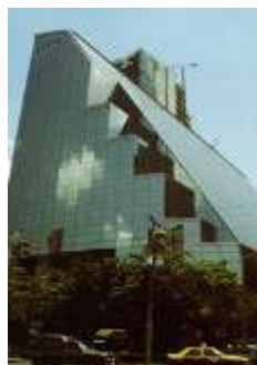
SIRIPINYO BUILDING - M,E -
